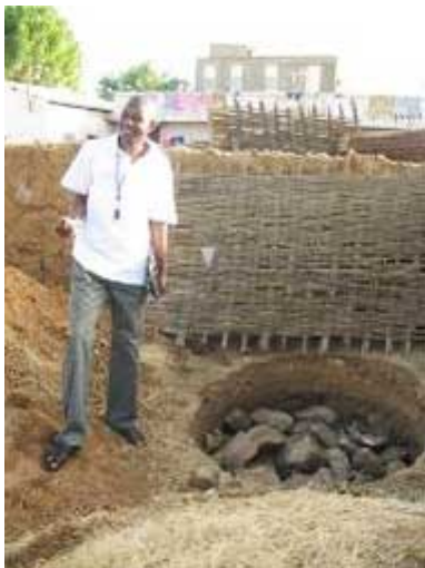
Filling a sump with pebbles in Mali.
