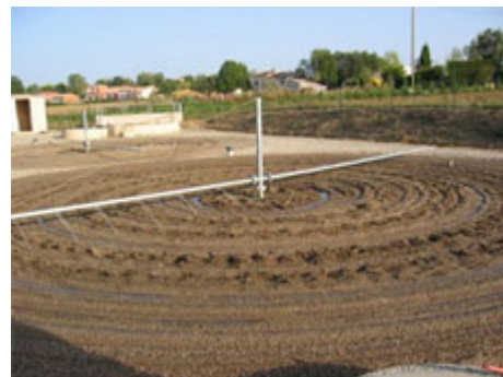
2) Filtering mass of the Mazens plant
