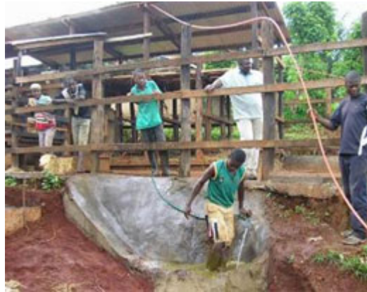
Filling a digester with diluted cow dung in another Biogas project in Africa. Photo Eric Florantin Tankeu
