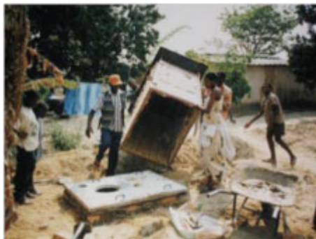
Installing or transferring a lightweight superstructure Photo by CREPA
