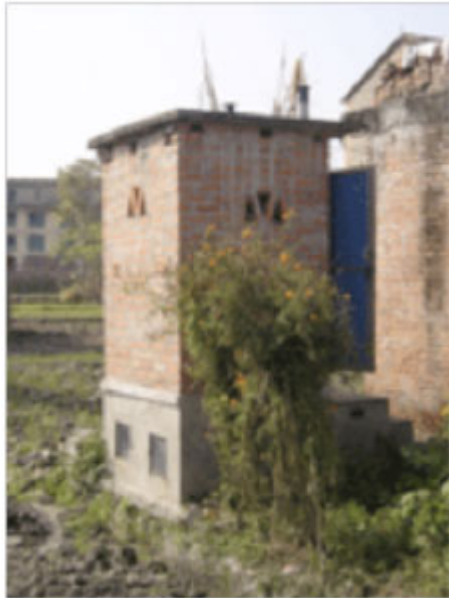
Latrine with two raised pits Photo by WELL
