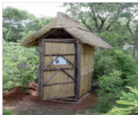
Simple removable structure Photo by CREPA
