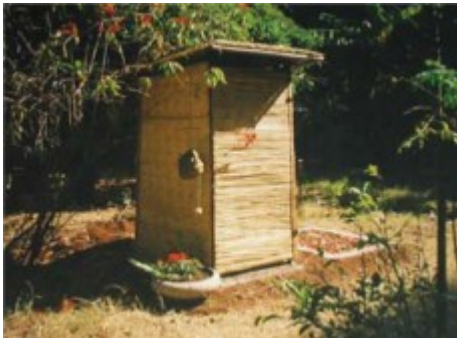
Twin-pit latrine with a lightweight, moveable structure - Photo CREPA
