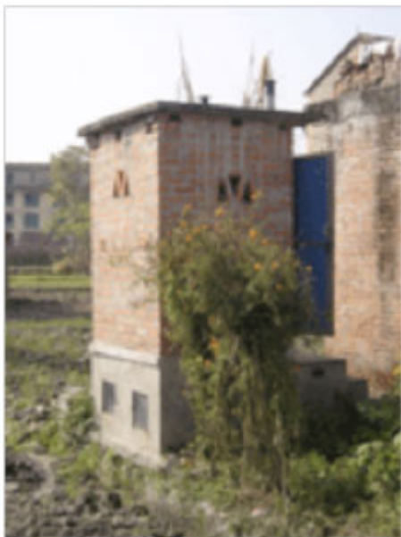
Latrine with two raised pits
