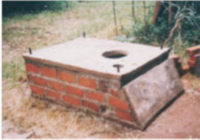
Manufacturing of a slab and a compartment. Photo by CREPA
