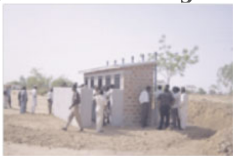
Public latrine in Nigeria. Photo by WEDC
