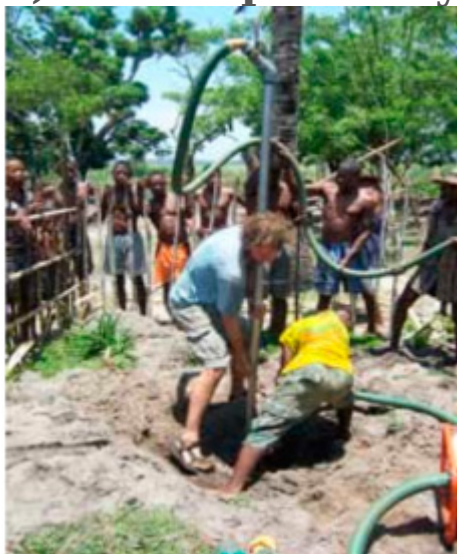
Drilling a well in Madagascar using the jetting method - Photo PS Eau 📷
