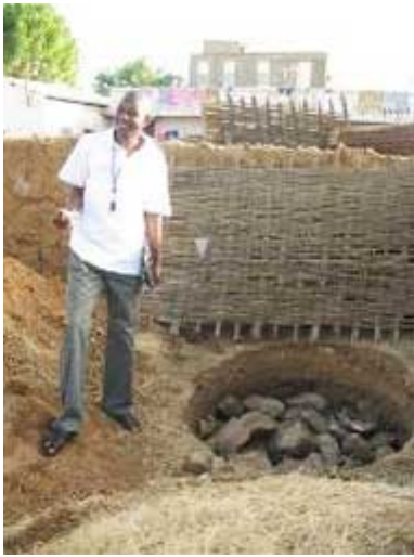
Filling a sump with pebbles in Mali. Photo PSEau
