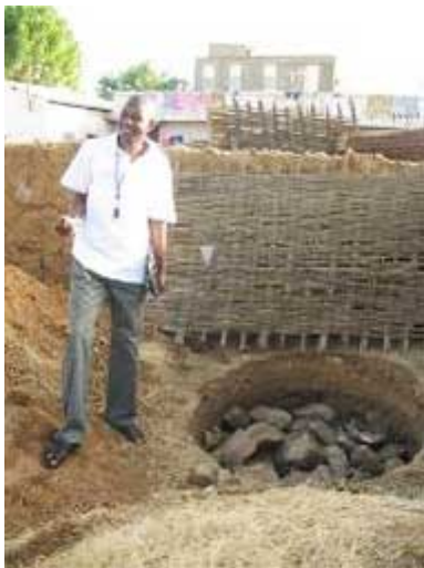
Filling a sump with pebbles in Mali.
