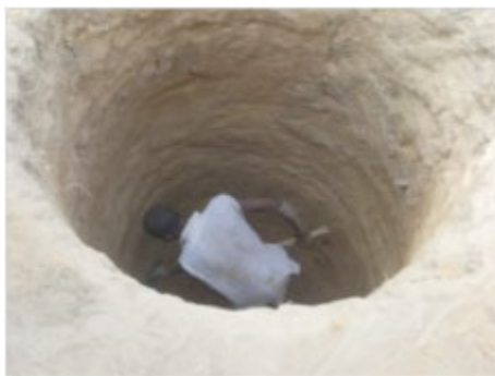
Digging a large sump in Mali. Photo PSEau
