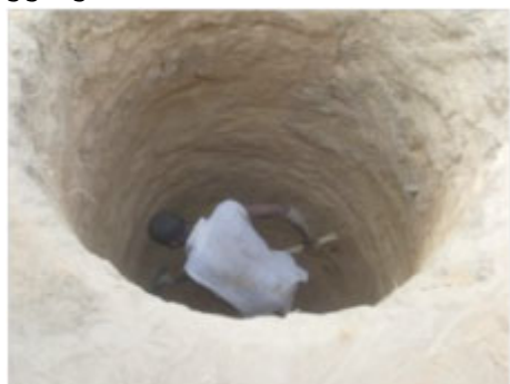
Digging a large sump in Mali. Photo PSEau
