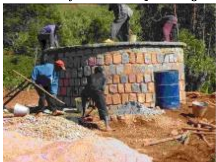
Building a stone reservoir
