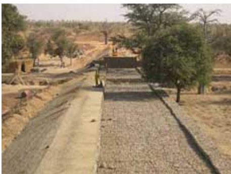
Construction of a dam in Mali (photo HSF)
