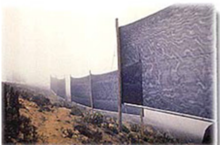
Fog collectors in El Tofo, Chile. Ph.Journaldunet
