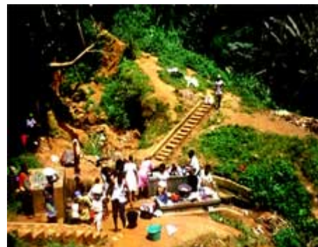
Spring catchment and fitting out with washing areas at Yaoundé (Cameroun) (Photo C.Le Jallé PSEau)
