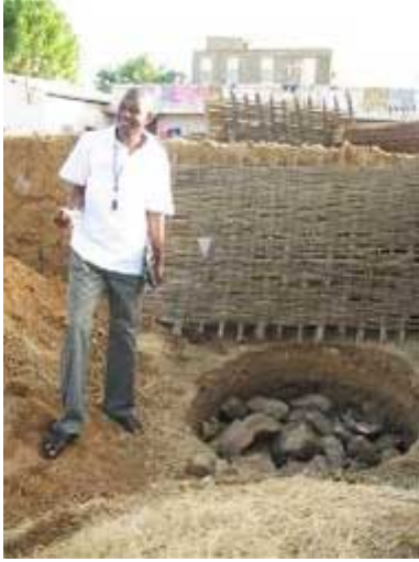
Filling a sump with pebbles in Mali.
