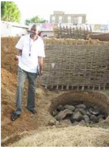
Filling a sump with pebbles in Mali.
